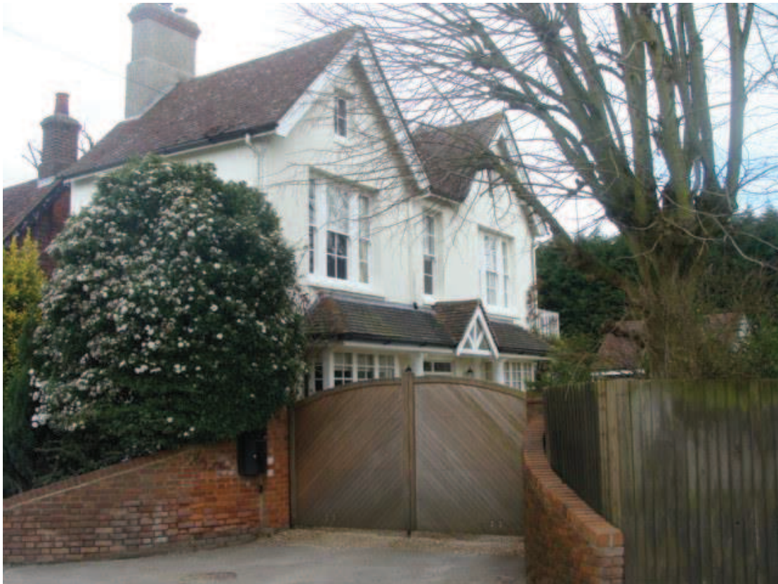
Picture 9. The Limes a residential building of quality and a strong feature in the local street scene.
