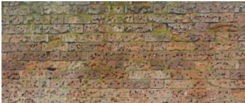
Picture 28 and 29. Detail of fine walled garden to north of Garden House. The decorative wooden gate is now bricked up behind. It previously provided access through to Culverwood House. Note central statue and remains of iron arches. Lower picture shows wall pockmarked by supports for fruit trees whose branches were pinned to the brickwork.
