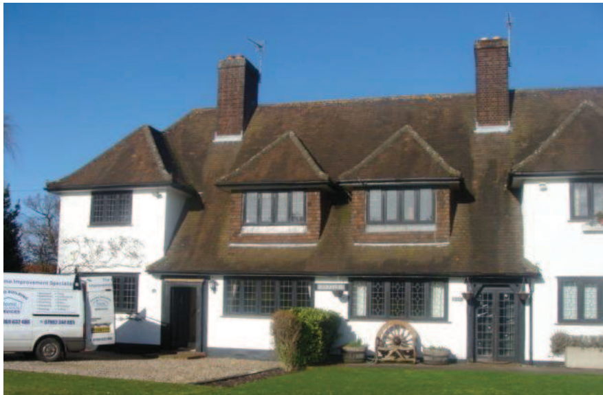
Picture 12. Nos. 20-21 Brickendon Green. First shown on mapping dating from the 1920's. These early 20th century properties with their steep roofs and prominent chimneys are prominent in the street scene and worthy of retention.
