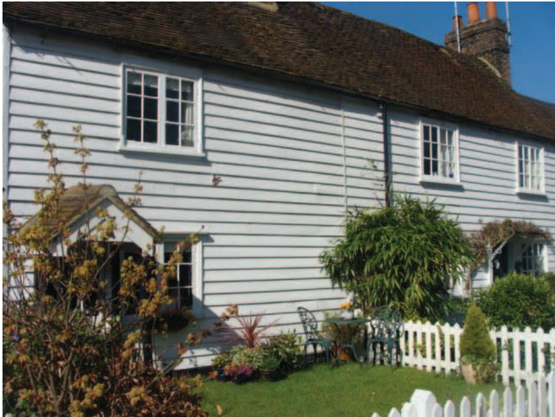
Picture 3. Nos. 6-8 Church Road Simple listed weather boarded cottages with tiled roofs.
