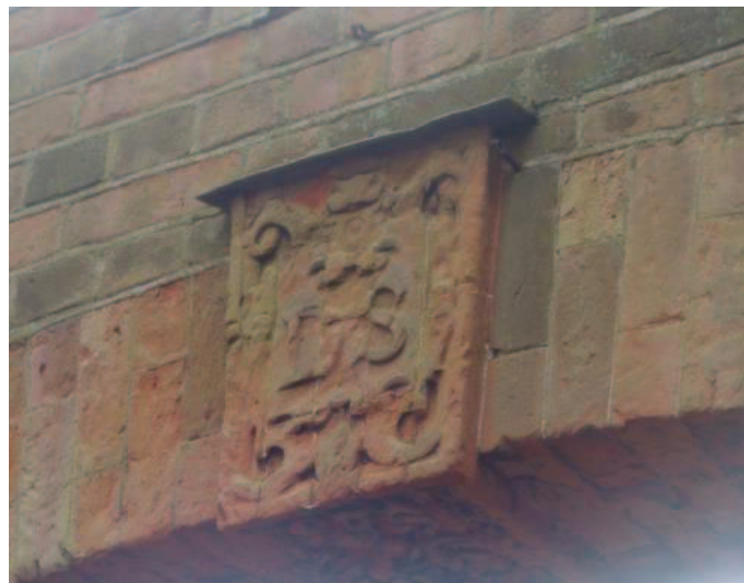
Pictures 23 and 24. Prominent garden walls of considerable architectural merit and historic importance south east of Fanshaws mansion and in good condition.
