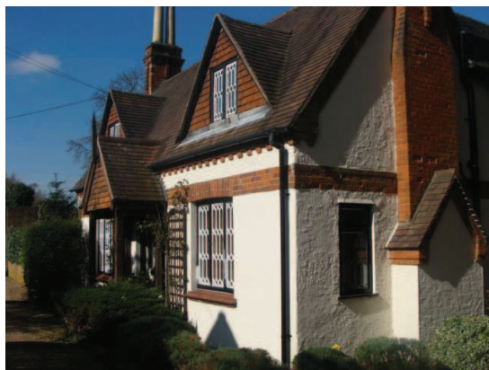
Picture 11. Wall House Cottage, although extended significantly this building in part displays features worthy of additional protection.
