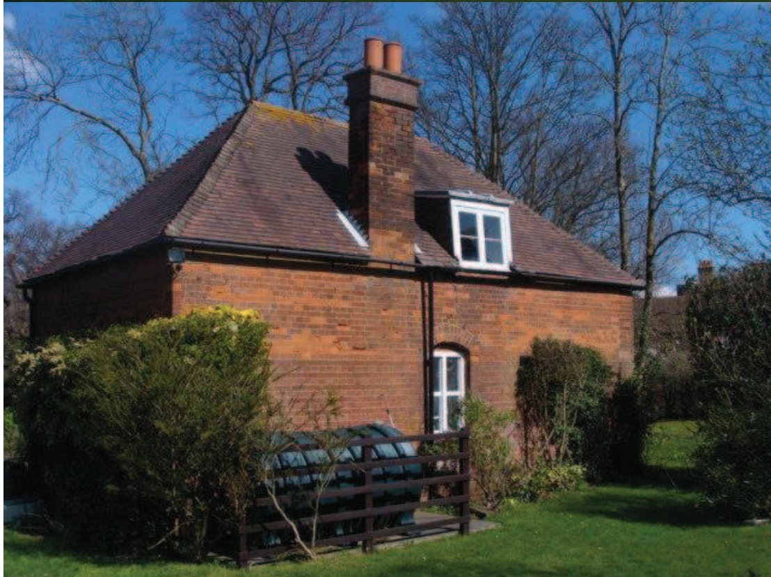
Picture 13. Trewinnard and outbuilding being formerly the Vicarage. A handsome building most worthy of retention with a number of high quality architectural features. The owner advises windows to front elevation are like for like replacements which represents best conservation practice.
