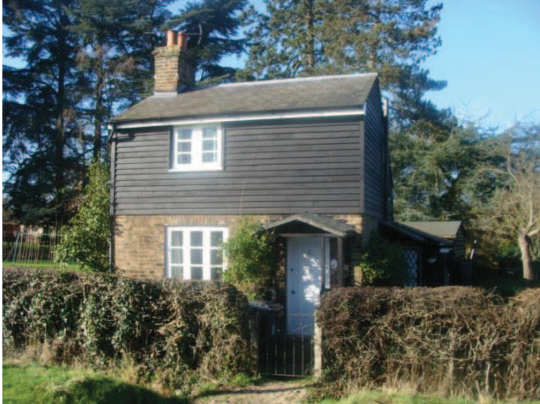
Picture 18. No 33 Brickendon Lane a small and unusually designed residence, worthy of retention.
