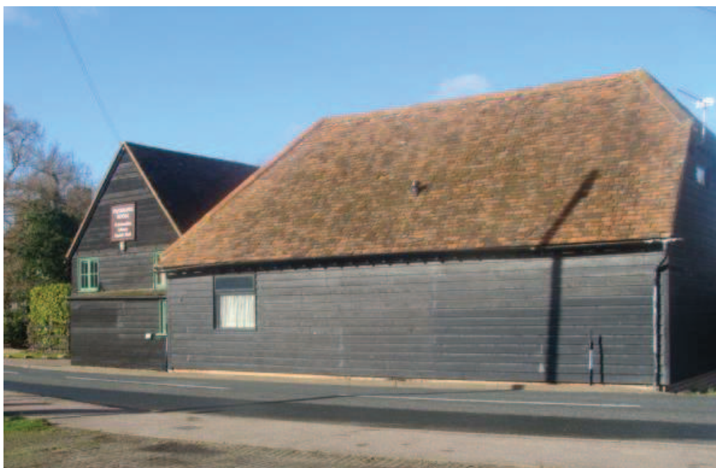
Picture 6 - The village Hall, a successful conversion of to the left - and former agricultural barn. Their success in part has been achieved by limiting the numbers of openings and retaining traditional materials.
