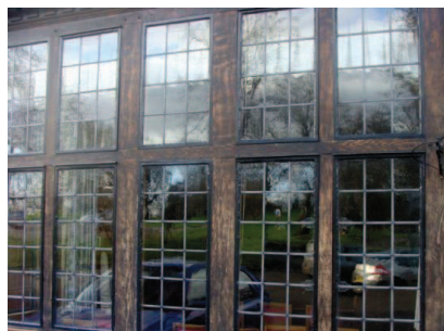
Picture 8. Fine window detailing at Brickendon Grange Golf Club.
