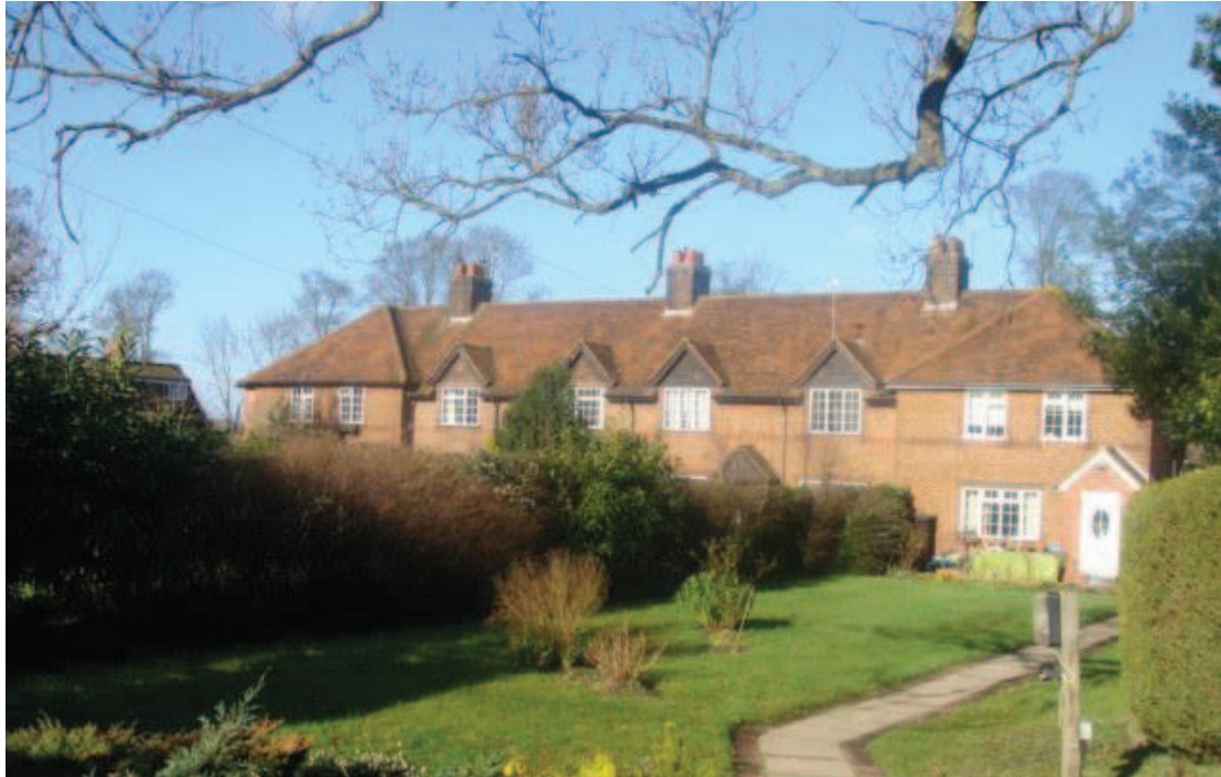
Picture 14. Nos. 5-11 Brickendon Lane - a mid 20th century terrace set back from the road with selected features most worthy of retention and additional protection.
